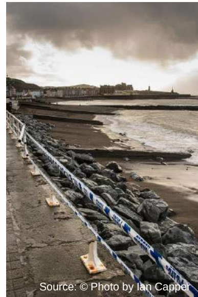
damaged railings near a beach
