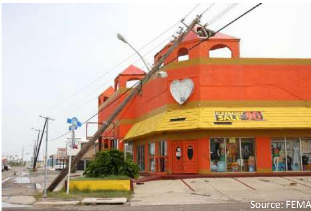
power-cuts because of damaged power lines
